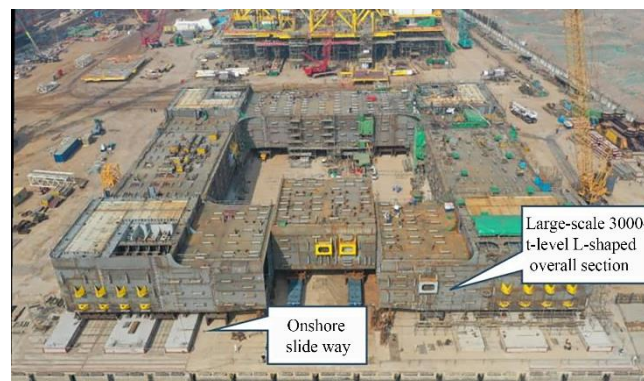
Fig. 8. Assembly on slideway of hull large-scale L-type overall section.
