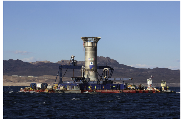
Fig. 8. Intake structure being lowered into position.
