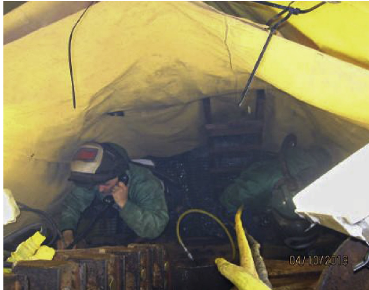
Fig. 6. Cutterhead repair.
