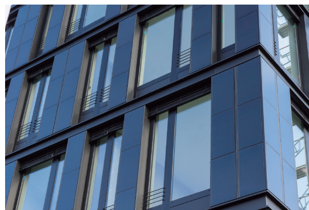
Fig. 8. CIGS modules as facade elements on the ZSW building in Stuttgart, Germany.
