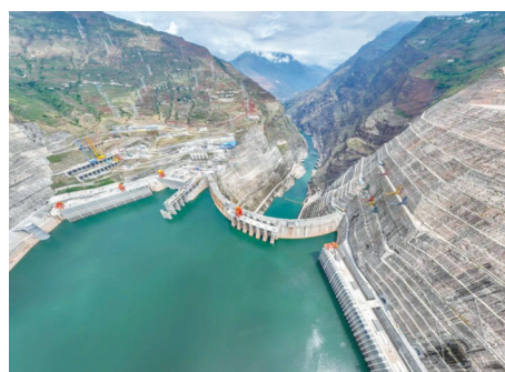
Fig. 2. The Baihetan Dam in June 2022 when it passed a 72 h trial and started formal operation of half its total complement of 16 Francis turbines, each with a generating capacity of 1 GW. When all 16 of these world's largest turbines are in operation, expected by the end of 2022, the dam will become the second-largest hydropower generator in the world. Credit: China Three Gorges Corporation (public domain).
