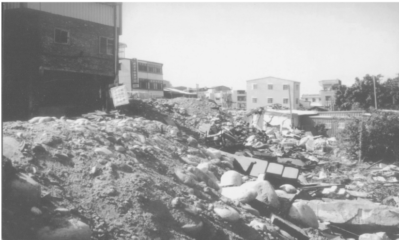
图 5 在断层上的房屋成了一片瓦砾，而其旁的楼房与平房相对完好 Fig.5 Houses on the fault turned to ruins, while those on the sides remained intact
