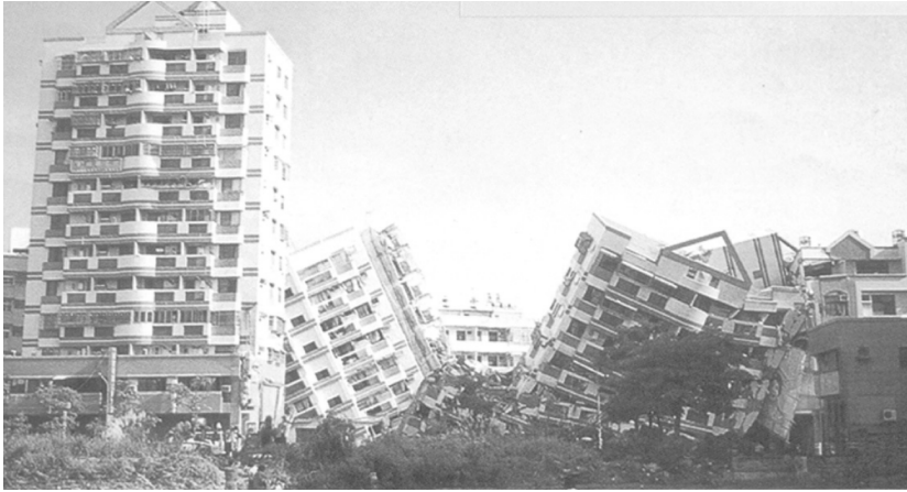
图 4 断层通过的地方，地形起伏同时也倾倒了部分建筑物 Fig.4 On the way that the fault passes through, the ground undulated and some buildings toppled over
