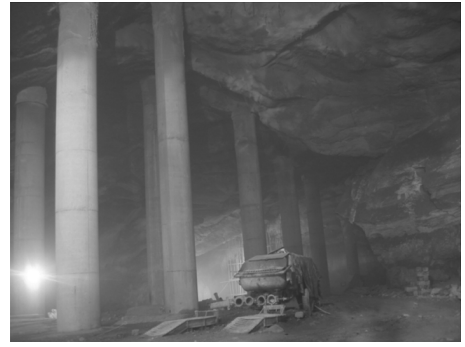
图9 溶腔大厅立柱支顶 Fig.9 Support pillar of caverns hall roof
