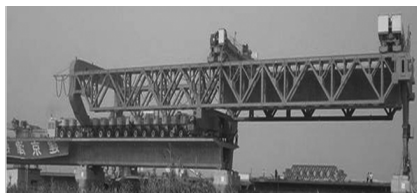
图 11 拼装式 SPJ900/32 型架桥机 Fig. 11 Assembling SPJ900/32 type bridge erecting machine
