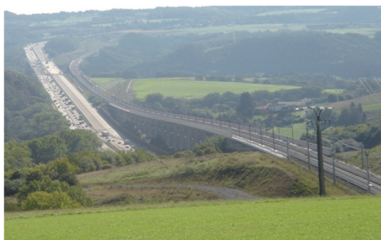
图3 某高速铁路典型平纵断面组合曲线 Fig. 3 Typical plan and profile section in high-speed railway
