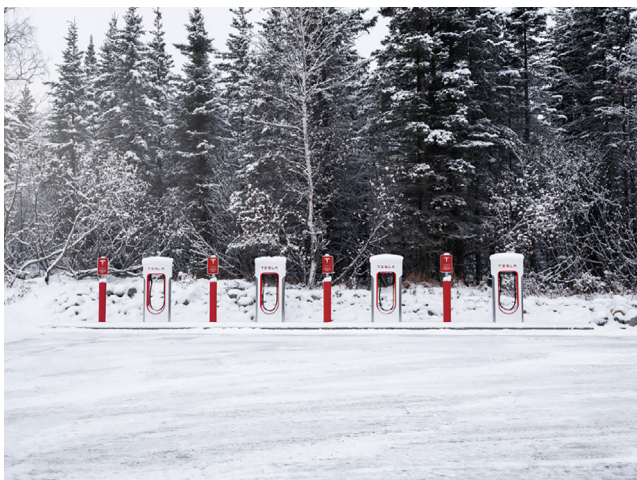
Fig. 1. A Tesla Supercharger station in the United States with four proprietary ports capable of charging Tesla vehicles at 250 kW. Before the end of 2024, Tesla plans to modify many of its US stations, like this one, so its ports can charge any EV, as they already do in Europe and China. Credit: Tesla, Inc. (public domain).
