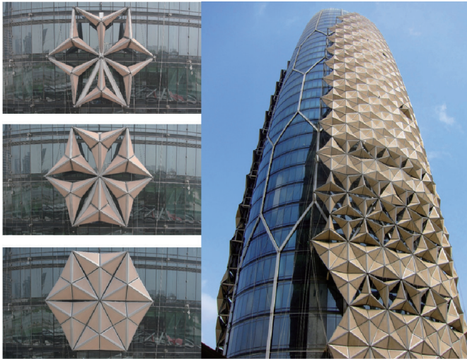
Fig. 2. Responsive building facades (Abu Dhabi).
