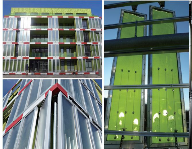
Fig. 5. The bioreactive facade—algae (Bio Intelligent Quotient (BIQ) House, Hamburg, opened April 2013)
