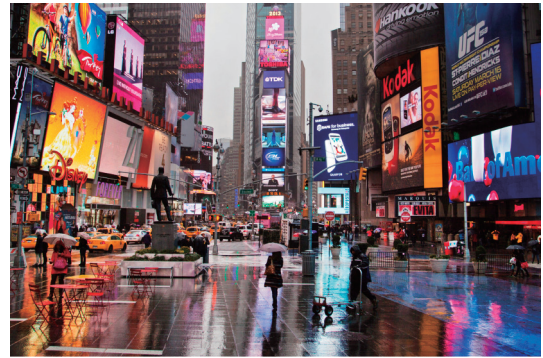
Fig. 13. Many cities around the world have centers that are predominantly media screens with advertisements, propaganda, and information. These types of facades require a considerable amount of energy and emit unnecessary heat during the time of day that should be reserved for cooling the city. (Available from: http://lssmedia.com/news/a-preview-of-cherry-blossoms-in-times-square/. )
