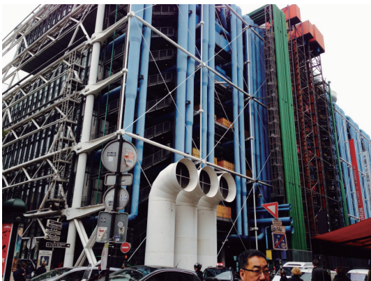
Fig. 11. The Pompidou Center by Renzo Piano and Richard Rogers was built in 1977. All of the structural and mechanical systems were exposed on the outside of the building and became part of the facade aesthetics. (Image courtesy of DOSU Studio Architecture.)
