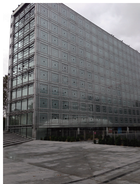
Fig. 14. The facade of Musée de L'Institut du Monde Arabe in Paris was an attempt to make a facade respond to the moving sun. (Image courtesy of DOSU Studio Architecture.)
