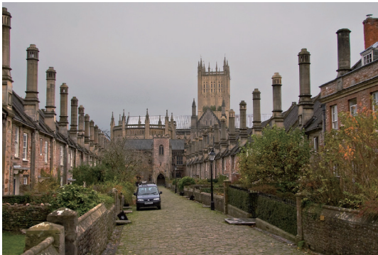
Fig. 10. Mechanical elements such as heating (chimneys) and other functional elements began to define the aesthetics of the facade in the Vicar's Close residential neighborhood in Wells, England in the mid-1300s. (Available from: http://gotterdammerung.org/photo/travel/england/wells/071121-155330%20Wells%20Cathedral%20Towers%20over%20Vicar's%20Close.html .)
