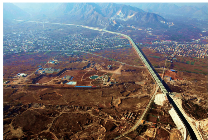
Fig. 3. The Cao River Aqueduct in the Middle Route Project (MRP).
