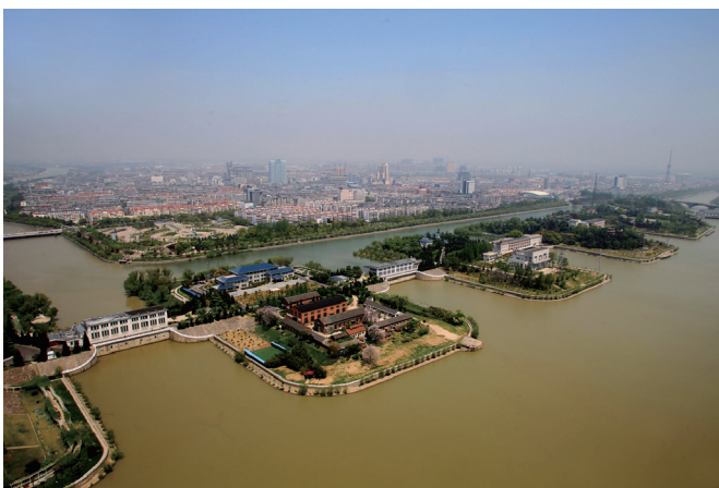
Fig. 2. Jiangdu Pumping Station in the East Route Project (ERP).
