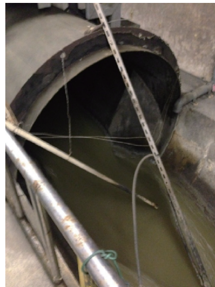
Fig. 2. Sewage pipe and sewage at the connection point Toyohashi 1.
