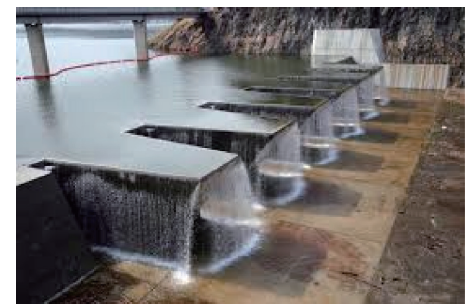
Fig. 7. Terminus fuse gates in the US.
