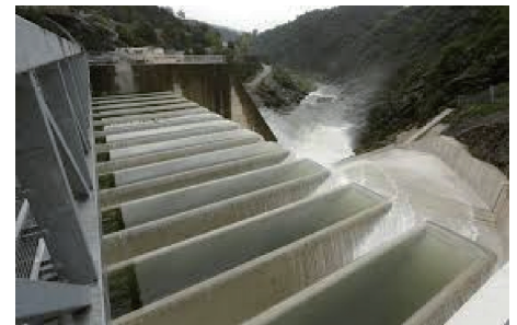
Fig. 4. The Malarce PK Weir in France.
