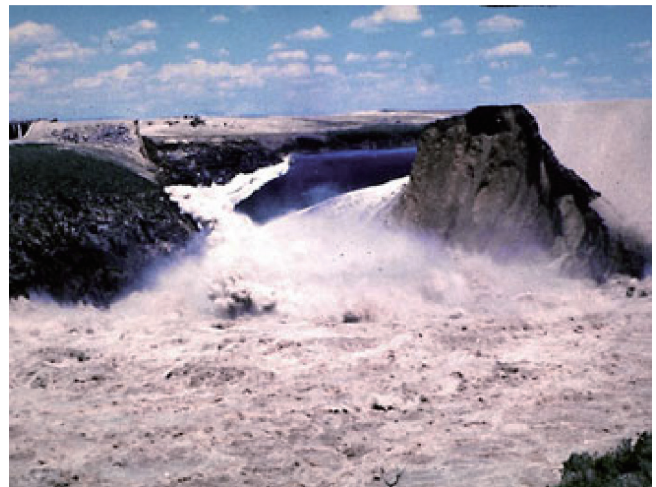
Fig. 9. The Teton Dam failure, 1976 (US).
