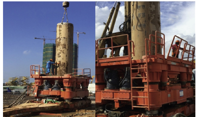
Fig. 5. Construction with an oscillatory casing drill.
