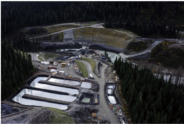
Fig. 6. ULR and construction water management facility at the upstream portal.
