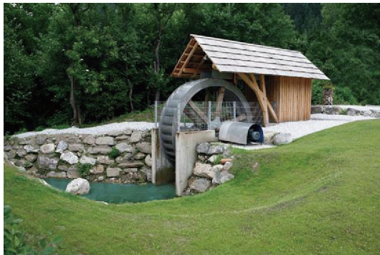
Fig. 3. Overshot water wheel, 4 m in diameter and 0.75 m wide.
