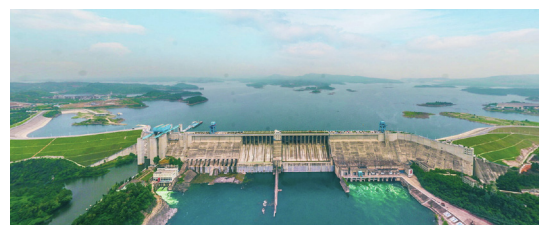
Fig. 2. The Danjiangkou Dam after completion of the heightening sub-project.
