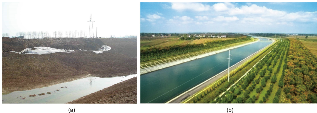
Fig. 5. (a) Expansive-soil landslides blocking the canals; (b) expansive-soil canals in the Middle-Line Project.
