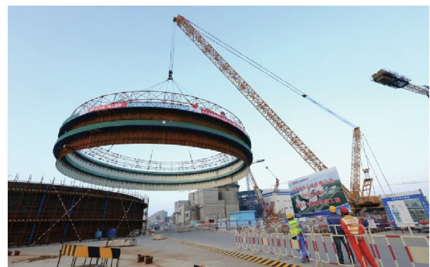
Fig. 9. Modular construction process of the steel lining for the containment of HPR1000.
