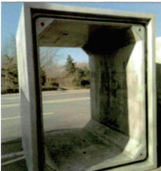
Fig. 3. Prefabricated concrete box culvert.
