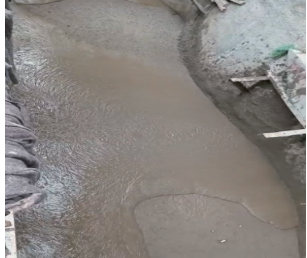
Fig. 16. Premixed solidified soil backfill.
