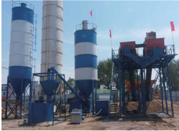
Fig. 15. Preparation and mixing system for premixed solidified soil.
