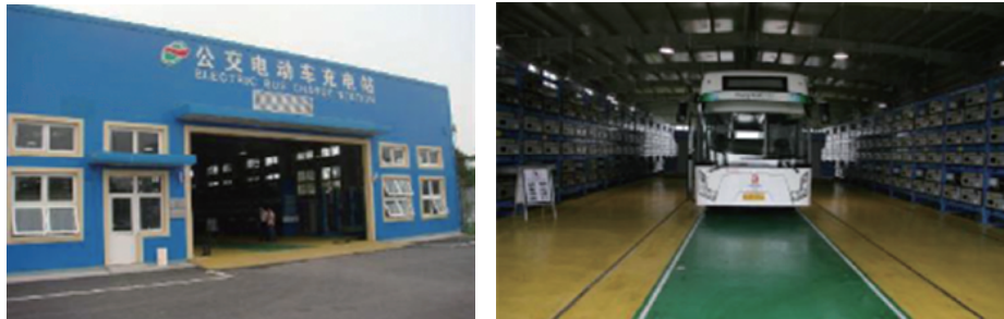
Fig. 7. Automated high-speed battery charging/swapping station for the Beijing Olympics.
