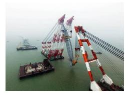
Fig. 7. Large-scale floating crane lifting a subsection.
