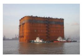
Fig. 2. Floating transportation of steel caissons.
