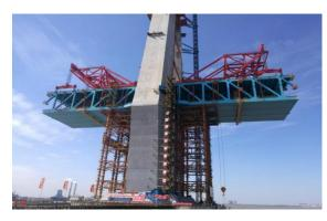
Fig. 8. Hoisting of double section Hutong Yangtze River Bridge girder.
