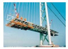
Fig. 10. Girder chip by girder crane.
