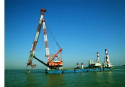
Fig. 5. Steel pile inserted by a barge.
