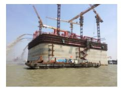
Fig. 3. Upper concrete caisson.
