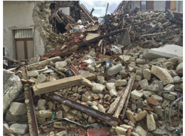
Fig. 3. Collapsed masonry buildings in the Amatrice earthquake in 2016.
