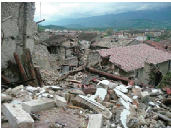
Fig. 2. Collapsed masonry buildings in the L'Aquila earthquake in 2009 [4].
