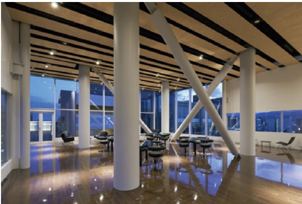
Fig. 17. A passively controlled building using BRBs (the Kyoto University of Foreign Studies).
