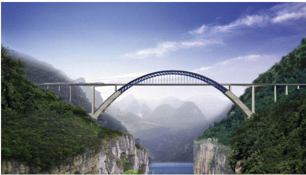
Fig. 7. Yachi River Bridge on the Chengdu–Guiyang High-Speed Railway.
