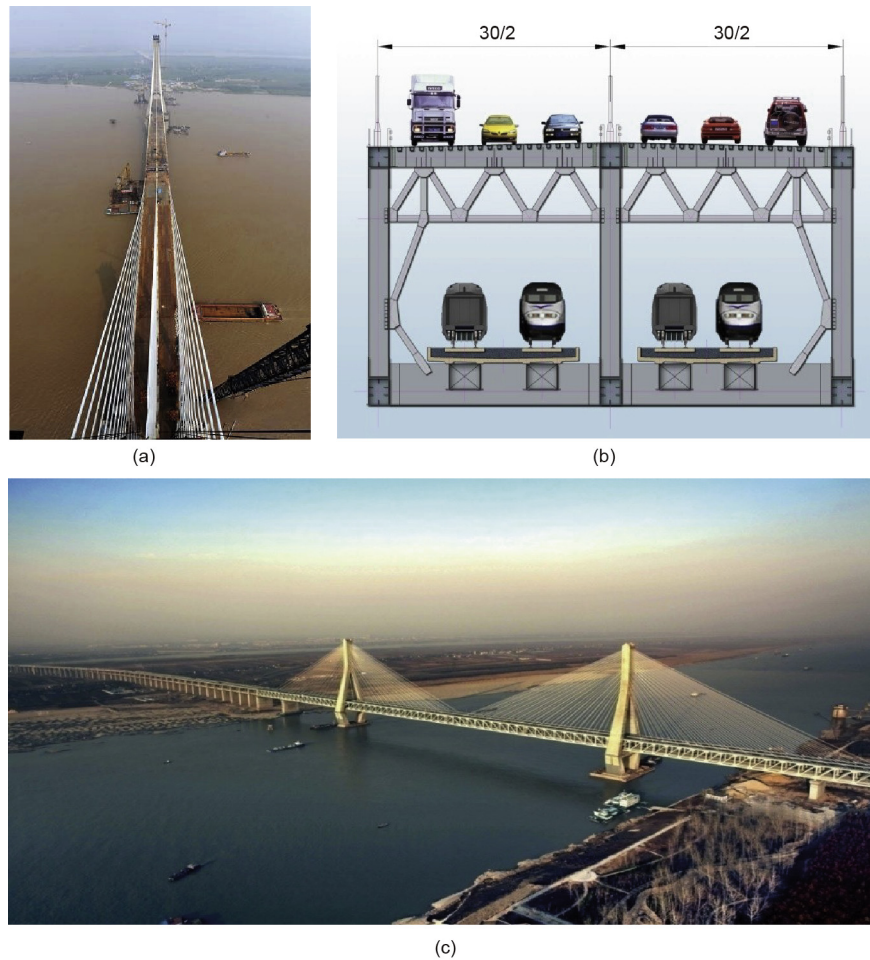
Fig. 2. Tianxingzhou Yangtze River Bridge in Wuhan. (a) Three cable planes; (b) layout of cross-section (unit: m); (c) constructed bridge.
