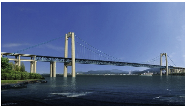
Fig. 3. Wufengshan Yangtze River Bridge.
