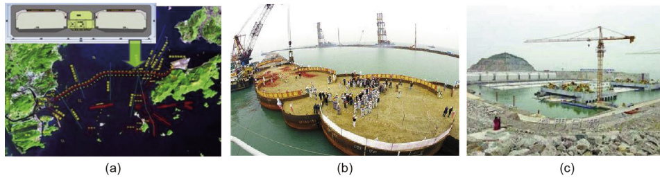
Fig. 15. (a) Plan layout for the immersed tunnel of the Hong Kong–Zuhai–Macao Bridge; (b) island cofferdam; (c) immersed tube transportation.
