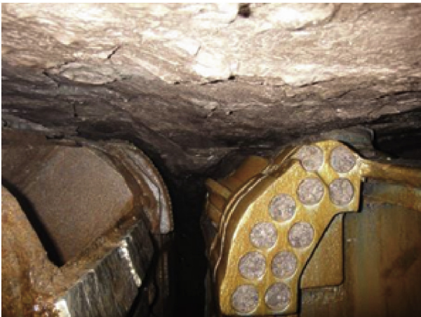
Fig. 9. The docking effect used in the construction of Shiziyang Tunnel.
