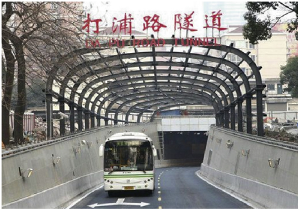
Fig. 1. Dapu Road Tunnel in Shanghai. †
