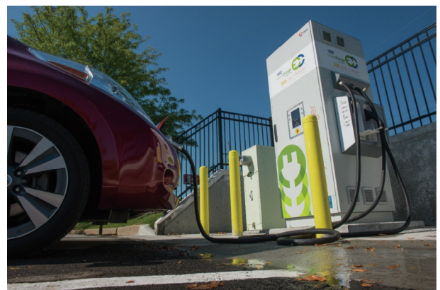
Fig. 1. A direct-current (DC) fast charger in Kansas City, Missouri, in the middle of the United States, recharges an EV’s battery. DC fast chargers deliver electricity at higher power and therefore charge vehicles more quickly than most other stations in charging networks. Of the 50 most populous US metropolitan areas, Kansas City stood out in a January 2019 EV industry analysis as the only one at the end of 2017 to already have enough chargers for its projected number of EVs in 2025. Credit: Evergy, with permission.
