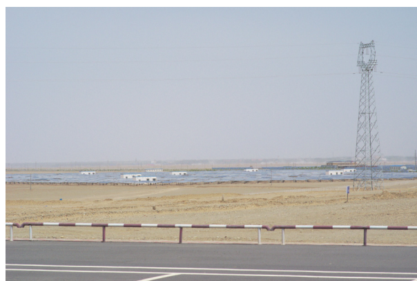
Fig. 1. A part of Gansu Dunhuang Solar Park, China's first solar energy generation facility, in the Gansu Province of western China. The area receives 3250 hours of sunlight per year and the Chinese State Council has set the goal of increasing Dunhuang's solar power generation capacity to 1 GW by 2020 from 50 MW in 2013. Credit: Popolon (CC-BY-SA-3.0).
