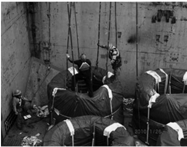
图9 起吊前准备 Fig. 9 Preparation before lifting
