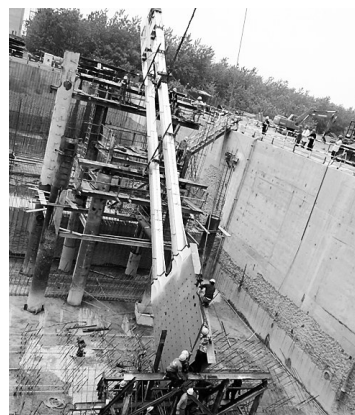
图11 锚固钢板现场安装定位照片 Fig.11 Anchor girder lifting photo
