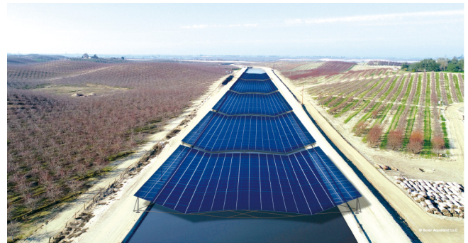
Fig. 1. An artist's conception shows what one of the canal-top solar arrays in California's Central Valley might look like after its completion in 2024. This section uses a canal-spanning truss design and will be 33 m across. Credit: Project Nexus (public domain).
