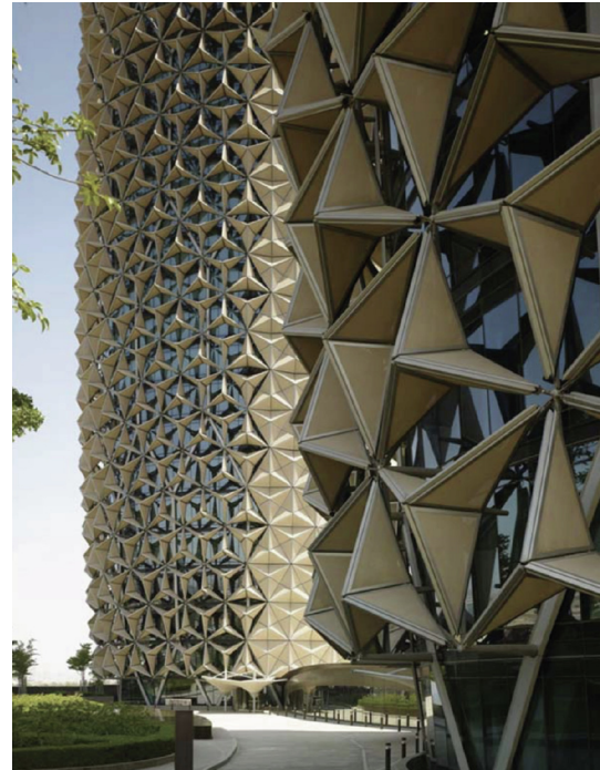
Fig. 1. Dynamic shading system of the Al-Bahr Towers. Reproduced from Ref. [11] with permission of the Creative Commons Attribution License CC BY 4.0, ©2015.
