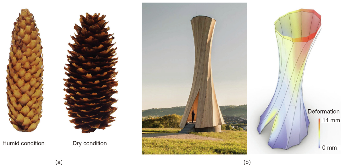
Fig. 5. Biomimetic design. (a) Spruce cones with different humidity conditions; (b) a self-shaping timber tower through moisture change. (a) Reproduced from Ref. [28] with permission of Elsevier, ©2017; (b) reproduced from Ref. [30] with the author credit “ICD/ITKE–University of Stuttgart”.
