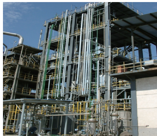
Fig. 3. A 10 kt·a -1 industrial demonstration unit of the gas-phase Beckmann rearrangement.
