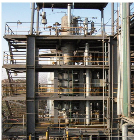
Fig. 7. The 6 kt·a -1 demonstration unit of the magnetically stabilized bed reactor.
