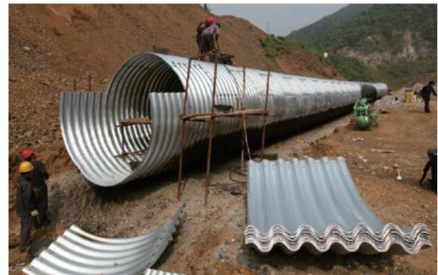
Fig. 5. Corrugated steel plate assembling picture.
