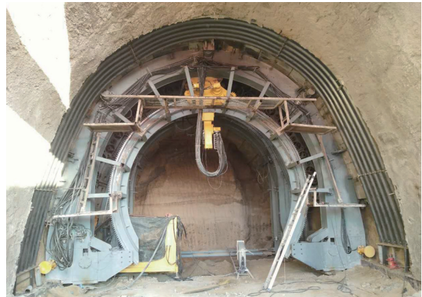
Fig. 4. Site construction of mobile supports.
