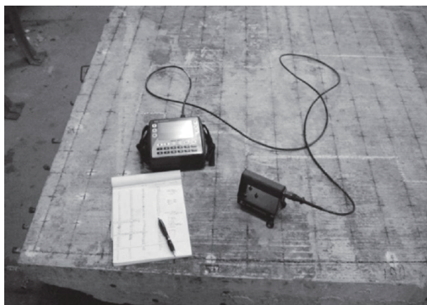
Fig. 4. Impact echo (IE) testing equipment.
