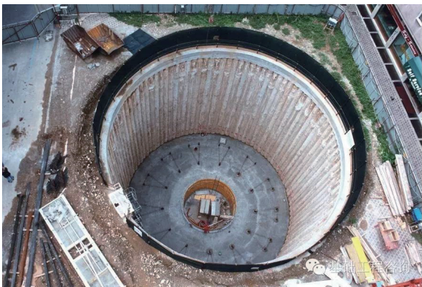
Fig. 12. “Pile-wall combination” cylindrical structure.
