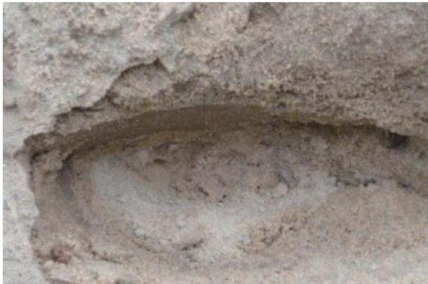
Fig. 6. Infiltration of sand fixing agent into the slope.
