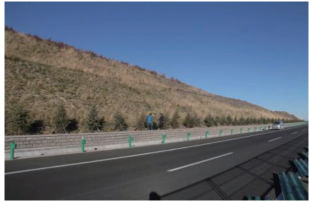
Fig. 7. Solidified effect of sand slope after two years.
