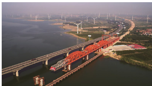
Fig. 12. Synchronous pushing for the construction of the Guanting Reservoir Bridge.
