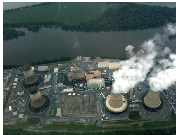
Fig. 1. This aerial photograph taken in 2010 shows the cooling towers of the Three Mile Island nuclear plant in Pennsylvania, on the Susquehanna River just south of the city of Harrisburg. In March 1979, the worst nuclear accident in US history left one reactor disabled and non-functional, Unit 2, on the left. Unit 1, on the right was unaffected by the accident but was decommissioned for economic reasons in September 2019, 15 years ahead of schedule. Credit: Wikimedia Commons (CC0).
