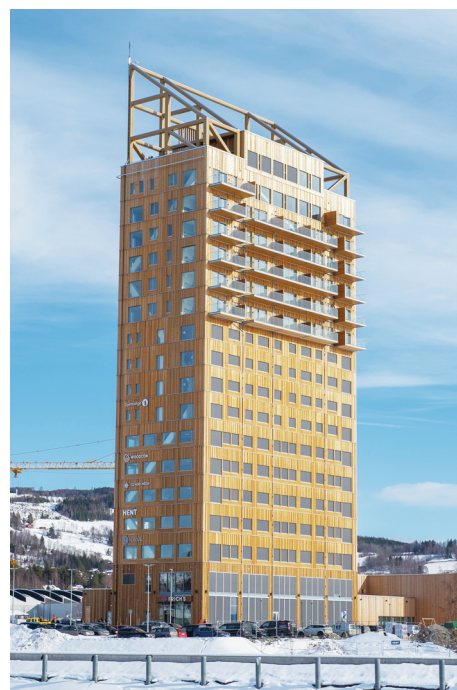
Fig. 1. The 18-story Mjøstårnet building in Norway gets most of its strength from engineered wood, which forms all its beams, columns, and trusses. The wooden beams that support its floors can be up to 720 mm thick, and the four columns at the corners of the building are 1425 mm thick. Credit: Wikimedia Commons (CC BY-SA 4.0).
