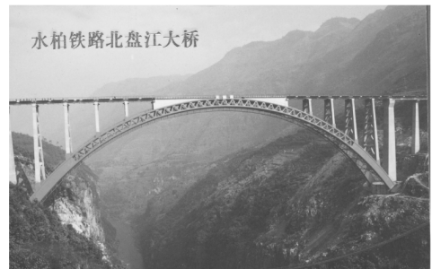
图 8 北盘江上承提篮式铁路拱桥 Fig.8 The type of carrying basket over deck railway bridge at Beipanjiang River
