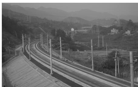
图 45 遂渝线无砟轨道试验段 Fig. 45 Experiment section of ballastless tracks on suiyu line
