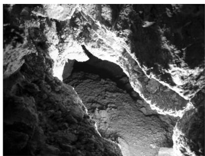
图 16 “+562”溶洞隧底空溶洞 Fig. 16 The empty cave of “+562” cave tunnel bottom
