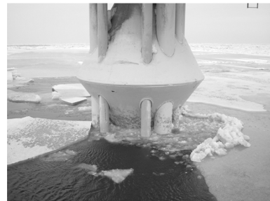
图 23 JZ9-3WHPB 平台破冰锥照片 Fig. 23 Photo of anti-ice cone on JZ9-3WHPB platform
