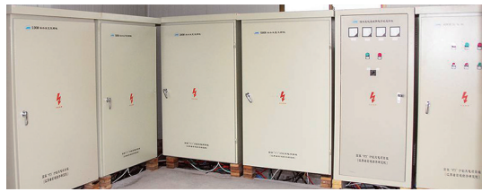
图1 非并网风/网智能协调供电控制器实物图 Fig. 1 The picture of non-grid-connected wind/grid intelligence controller
