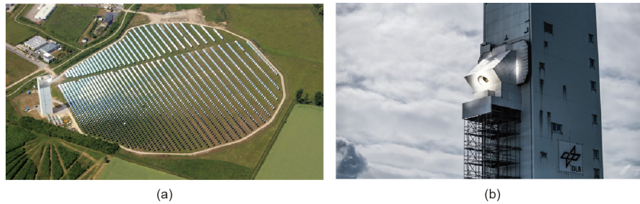
Fig. 8. DLR's experimental CSP plant: (a) Juelich Solar Tower and (b) particle receiver CentRec in test [66–68].
