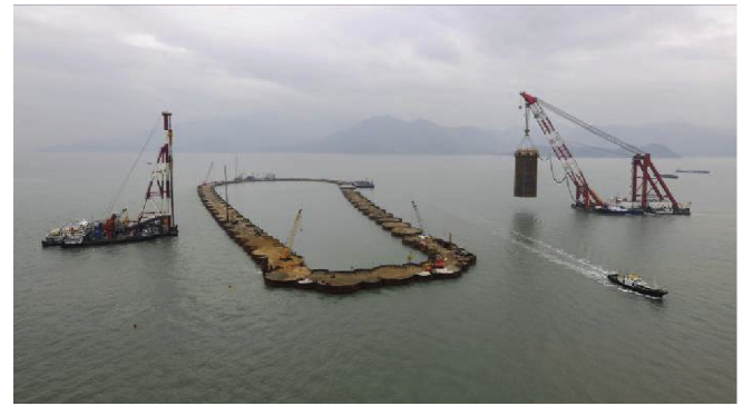
Fig. 3. The last cylinder to form the east island.
