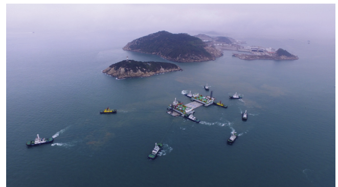
Fig. 7. Transportation of E30, the last element installed.
