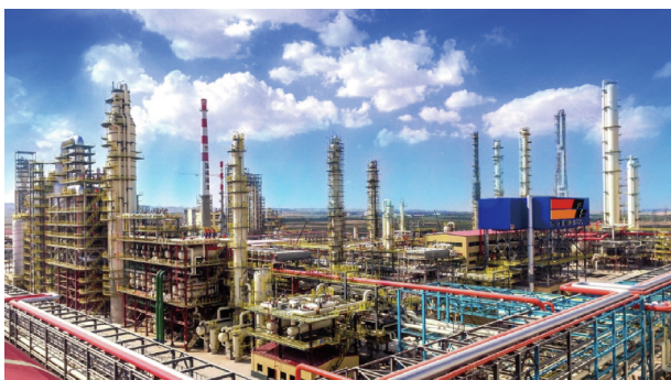
Fig. 3. The Baofeng Ningxia Phase II CTO plant, which was started up in 2018. With the use of the innovative DMTO catalyst, the consumption of methanol per ton light olefins in this DMTO unit is reduced to 2.85 t.
