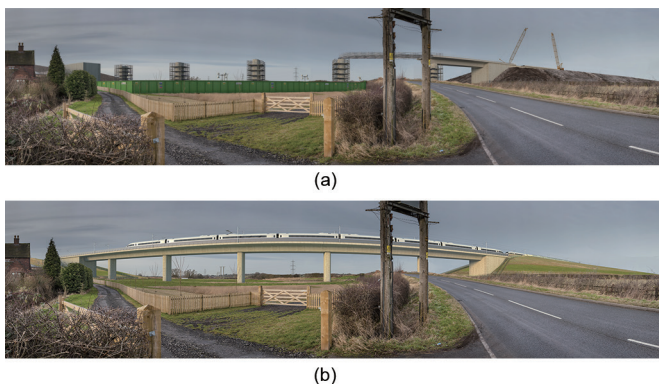
Fig. 2. The latest visualization technologies enable us to combine the wealth of available data to communicate the High Speed 2 scheme in visually accurate way. ©Arup.
