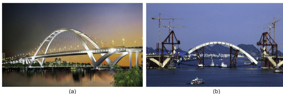
Fig. 7. Third Fenghuang Bridge. (a) Bridge after completion; (b) large-segment lifting of the main arch rib.
