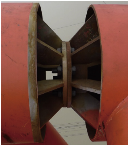
Fig. 11. Contact condition of the flange joint.
