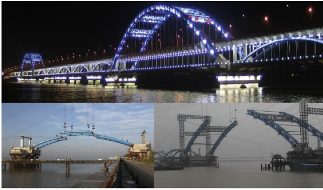
Fig. 5. Cable-stayed fastening-hanging cantilever assembly of Hangzhou Fuxing Bridge.
