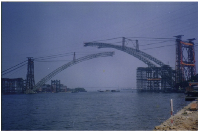
Fig. 6. Rotation construction of Guangzhou Yajisha Bridge.
