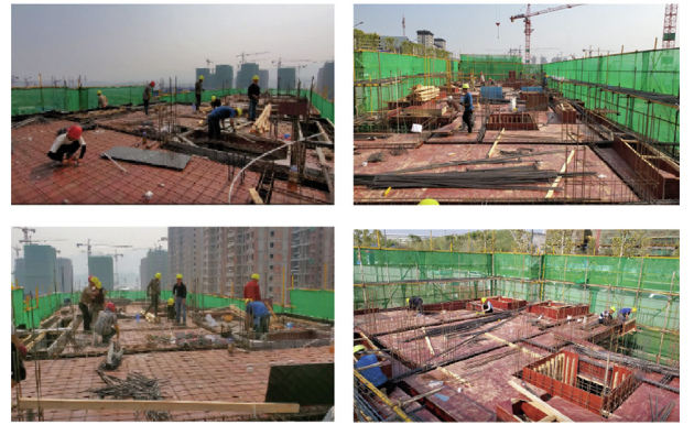
Fig. 8. Video frames of the construction scene.
